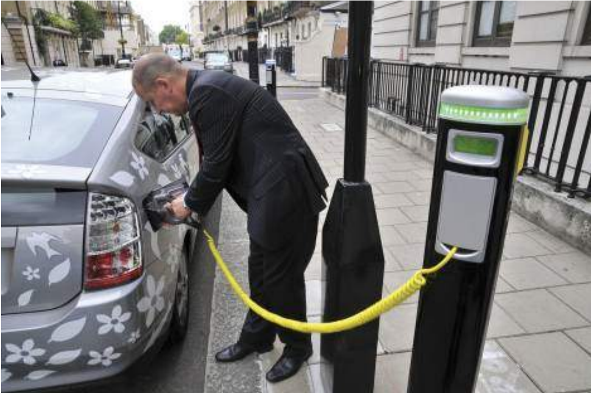
Figure 28. The San Francisco Bay Area has been expanding the number of EV charging stations rapidly. http://venturebeat.com/2010/08/10/bay-area-soon-to-be-home-to-5050-ev-charging-stations/
