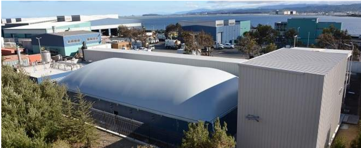
Figure 17. In partnership with Blue Line Transfer, Inc. – Sunset Scavenger has designed and developed the Blue Line Biogenic CNG (compressed natural gas) facility to produce over 100,000 diesel equivalent gallons of CNG per year. http://zerowasteenergy.com/what-we-do/our-projects
