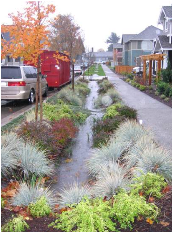
Figure 44. Green infrastructure such as bioswales are example to treat stormwater runoff. http://water.epa.gov/infrastructure/greeninfrastructure/what.cfm
