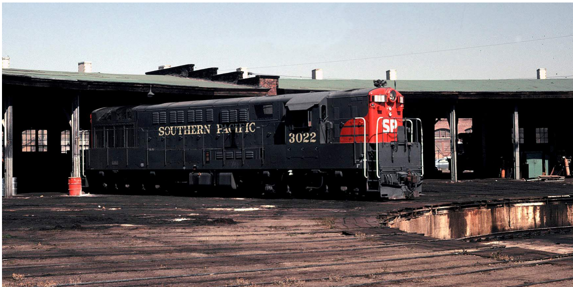
Figure 50. Brisbane Bayshore Roundhouse in need of restoration and revitalization. http://shawnclover.com/2011/11/05/the-old-abandoned-bayshore-roundhouse/
