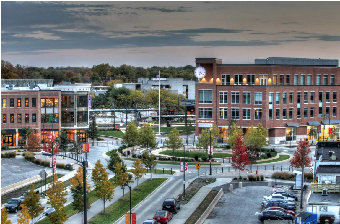
Figure 23. Multimodal uptown station in Normal, Illinois spurred impressive growth in transit ridership and mixed-use private downtown investment. http://bettercities.net/article/multimodal-station-and-plan-spur-town%E2%80%99s-revival-21378
