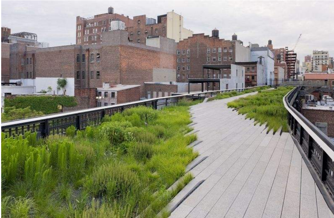
Figure 53. The Hudson Yards project located at New York City's railyard and its neighbor, the Highline Park project, are both milestones in sustainable building, adaptive reuse. Hudson Yards also features a pneumatic vacuum waste elimination tube system.
