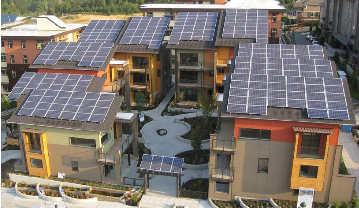
Figure 10. ZHome in Issaquah, Washington – Townhome project designed to achieve Zero Net Energy, as well as a number of other environmental benchmarks, which will become affordable housing in 2016. http://living-future.org/case-study/zhome
