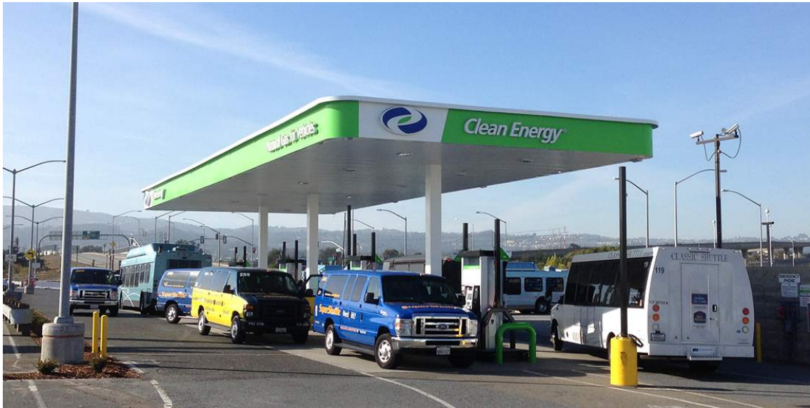
Figure 27. City of Brisbane currently does not have a gas station. Consider, in partnership with Recology's operations, providing CNG fueling.
